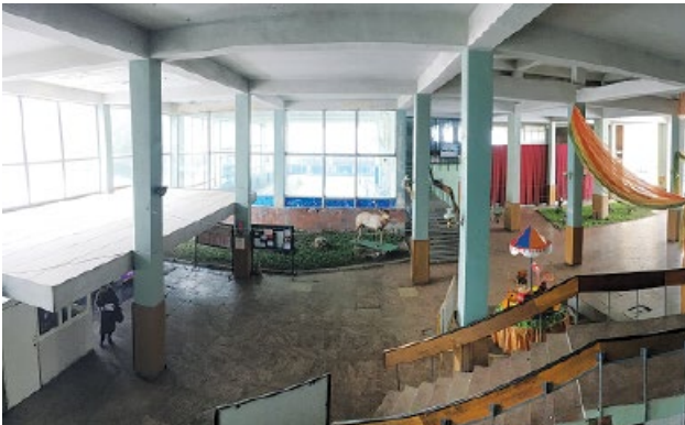
View of the lobby of the Erebuni youth and creativity center before and after retrofit.
