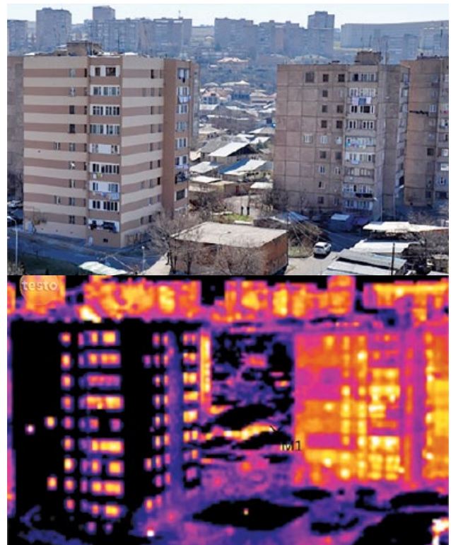
Energy efficient retrofitted residential building in Avan administrative district of Yerevan, next to similar non-retrofitted one. Same view with thermal imaging camera.
