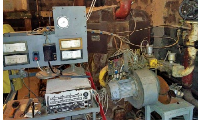
Boiler house before and after retrofit
