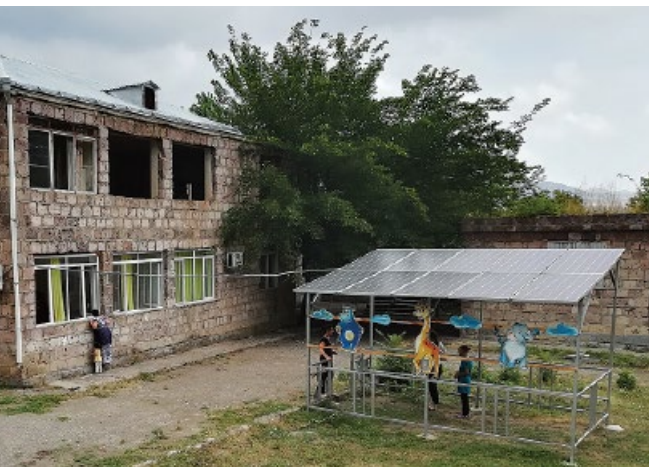
^ The installed solar panels in Berqaber near-border village kindergarten to exclude firewood based heating system
